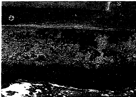
Figure 7. Exterior of CAL corresponding to rust stained region in Figure 6. Note horizontal crack above the water line level for unloaded vessel.
